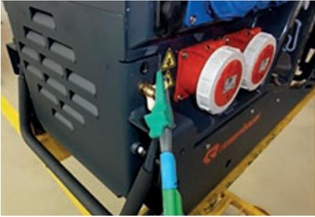
2. Measure contact resistance to PE contact for socket 1:
